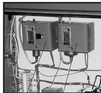
High pressurestat Figure 6.2I Low pressurestat
