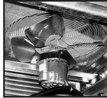
Typical fan assembly Figure 2.4A
