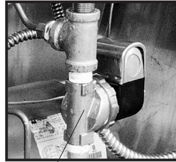
Typical water make-up solenoid valve Figure 5.4A
